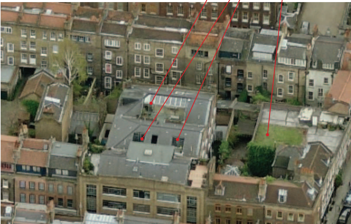
Figure 3: 6-10 Princelet Street viewed from the north
